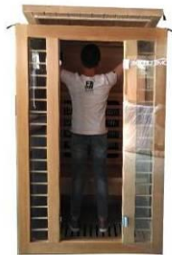
FIG-19 Setting the top panel
